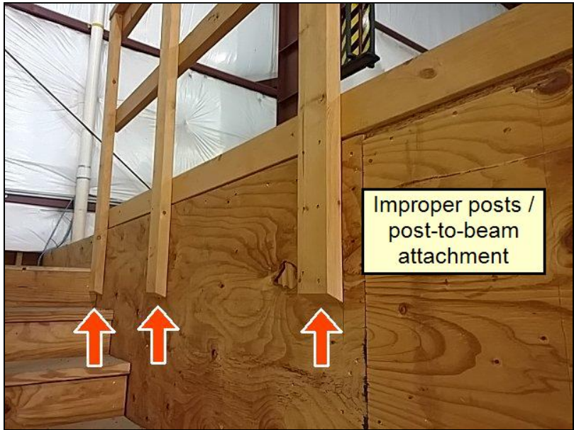
Loft guard rail attachment
